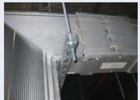
FO sensing cable secured into the fins of ventilated busbar using ordinary spring-loaded clip (i.e. office clip).
